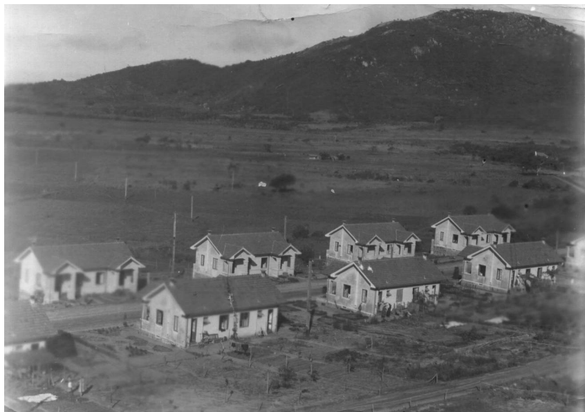
Figura 01: Vista do Hospital. S/d. CEDOPE.
